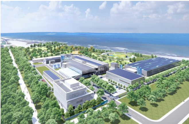
Hsinchu Sea Water Desalination Plant
