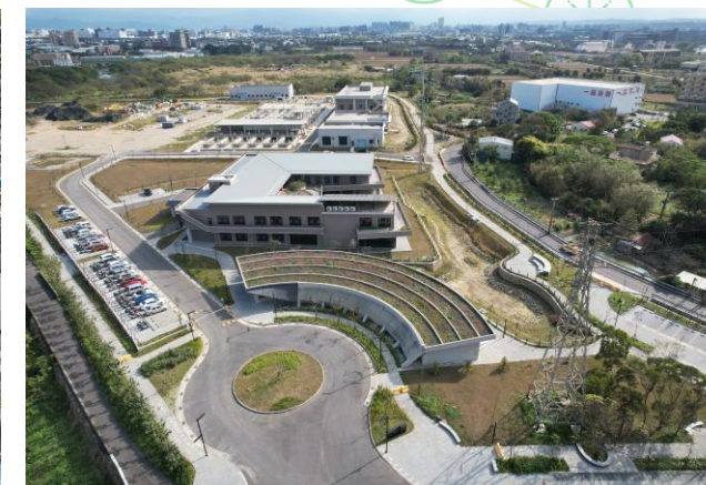
Zhongli Wastewater Sewer System
