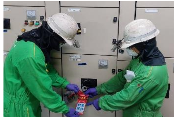
Electrical Equipment Isolation and Tagging Warning
