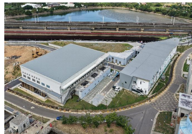
Taoyuan North District Water Resources Recycling Center
