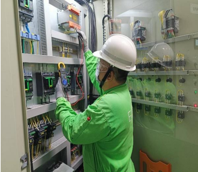
Power distribution panel inspection
