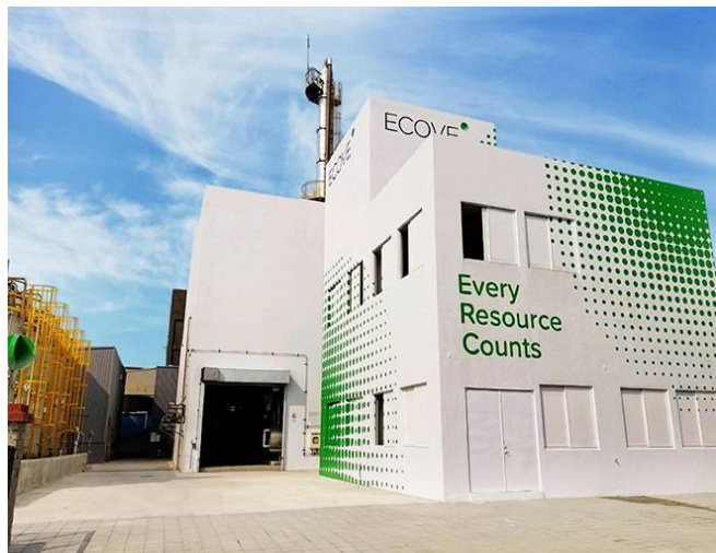
Solvent Recycling Plant
